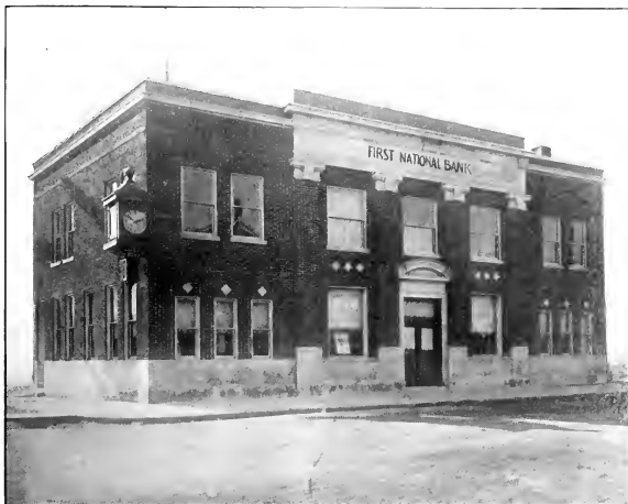
First National Bank, O'Fallon
